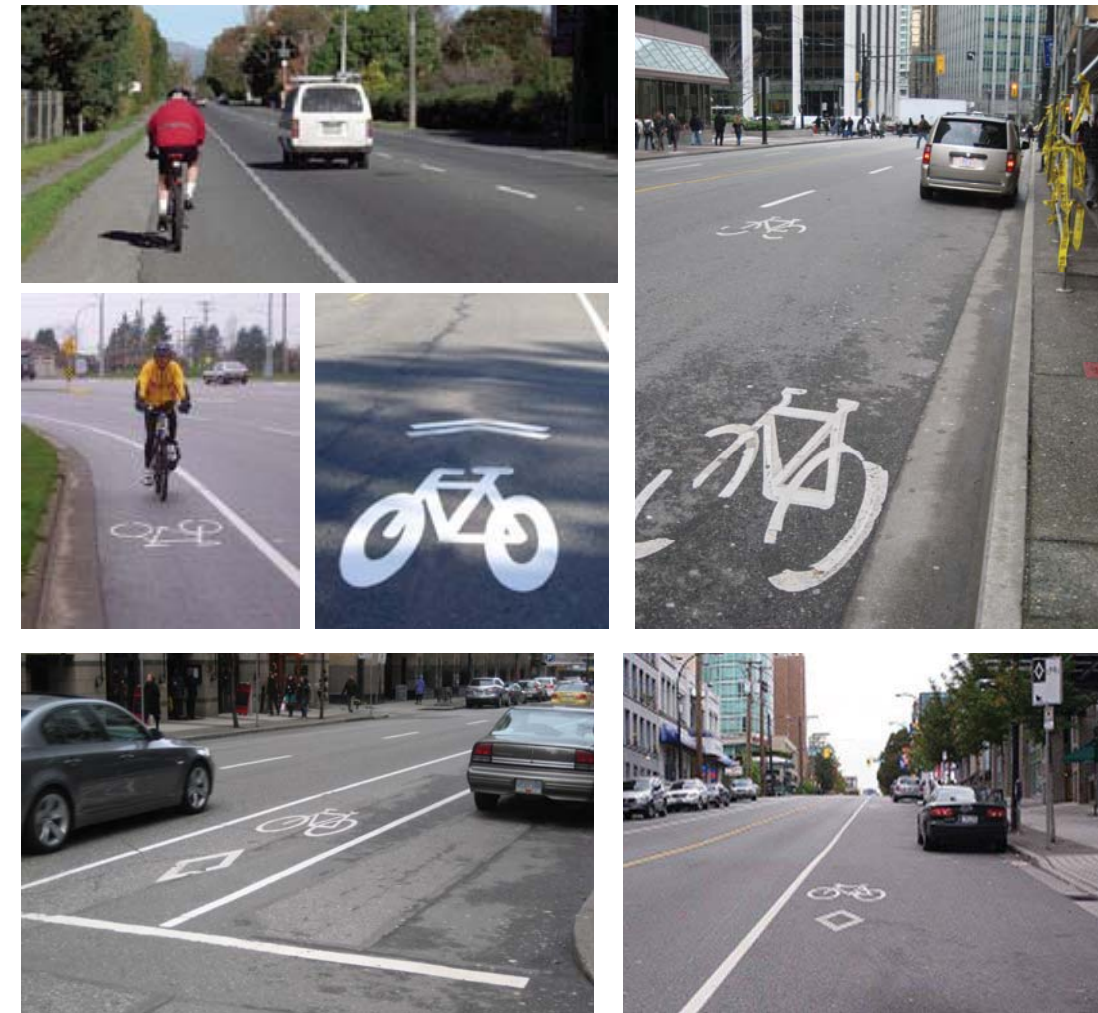
Figure 10.6: Examples of Pavement Markings.
