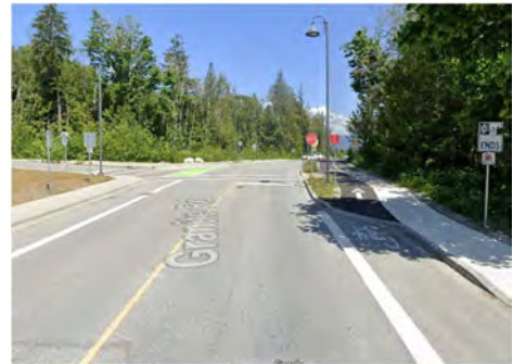
Figure 4: View of Derby Road
