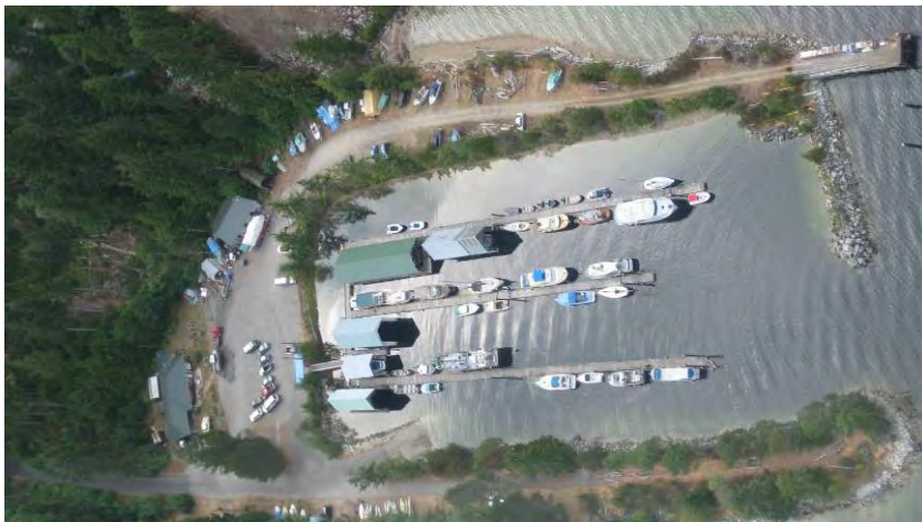
Marinas are important economic activities, providing access to marine areas for residents and visitors. Careful design and siting is needed to prevent impacts to water and shoreline ecology (Tillicum Bay).
