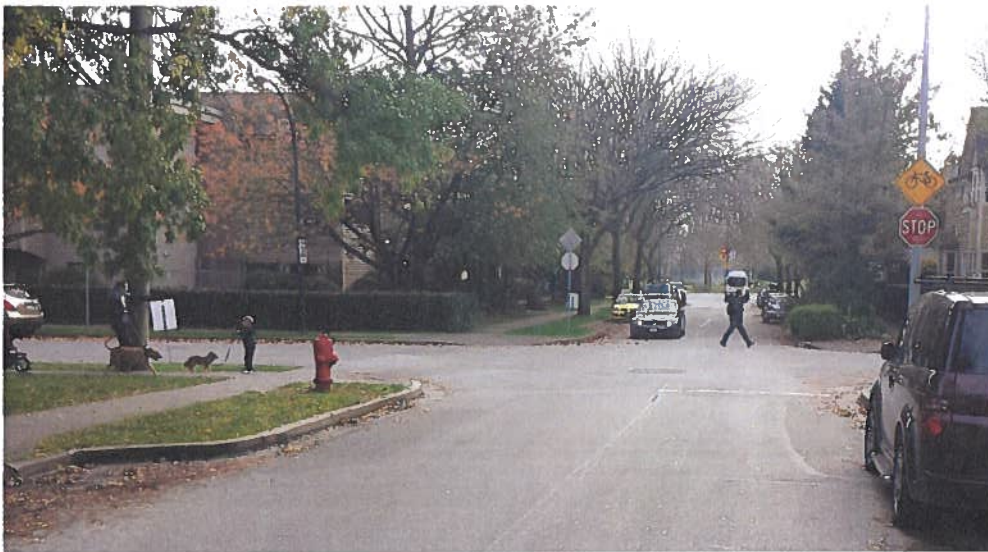
Figure 6.4: Example of Curb Bulge
