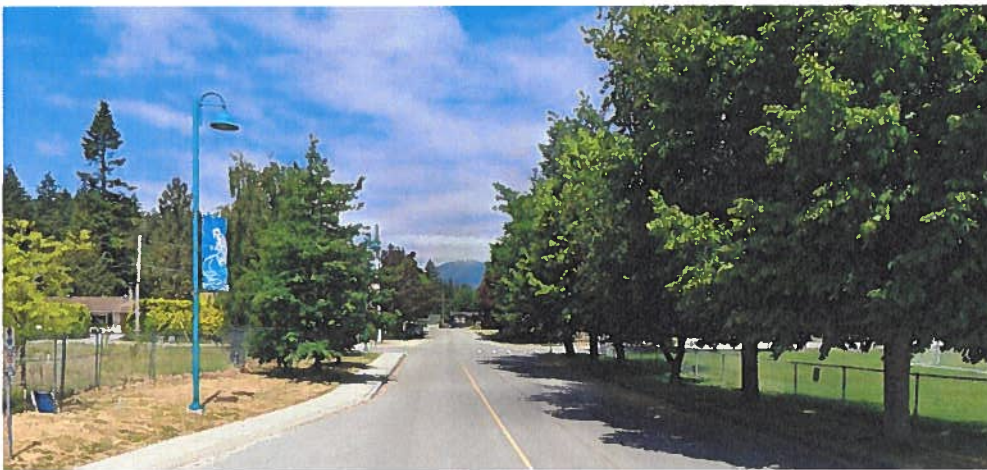
Figure 6.1: Northbound View on Ocean Avenue Approaching Medusa Street
