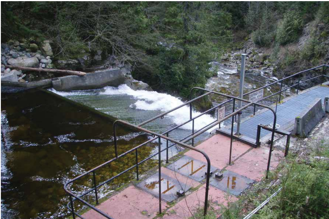
Photo 3 Chapman Creek SCRD Water Intake
