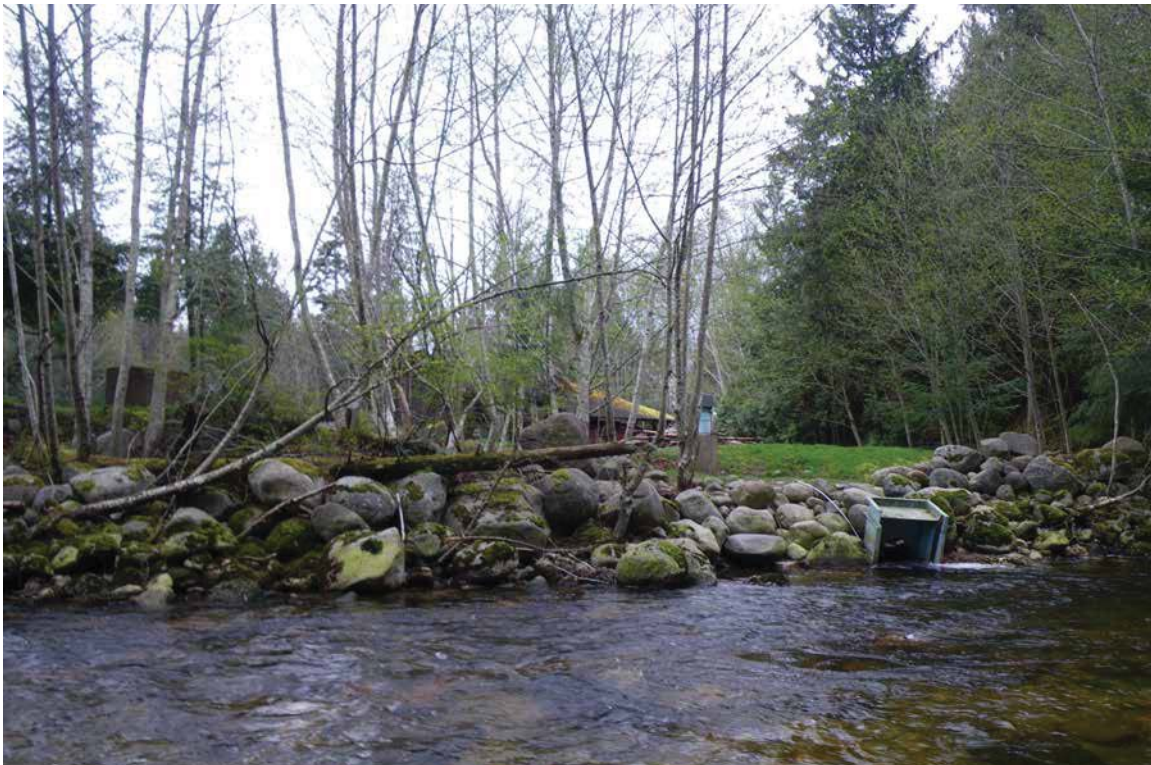
Photo 7 Informal bank protection works and intake structure at DFO hatchery
