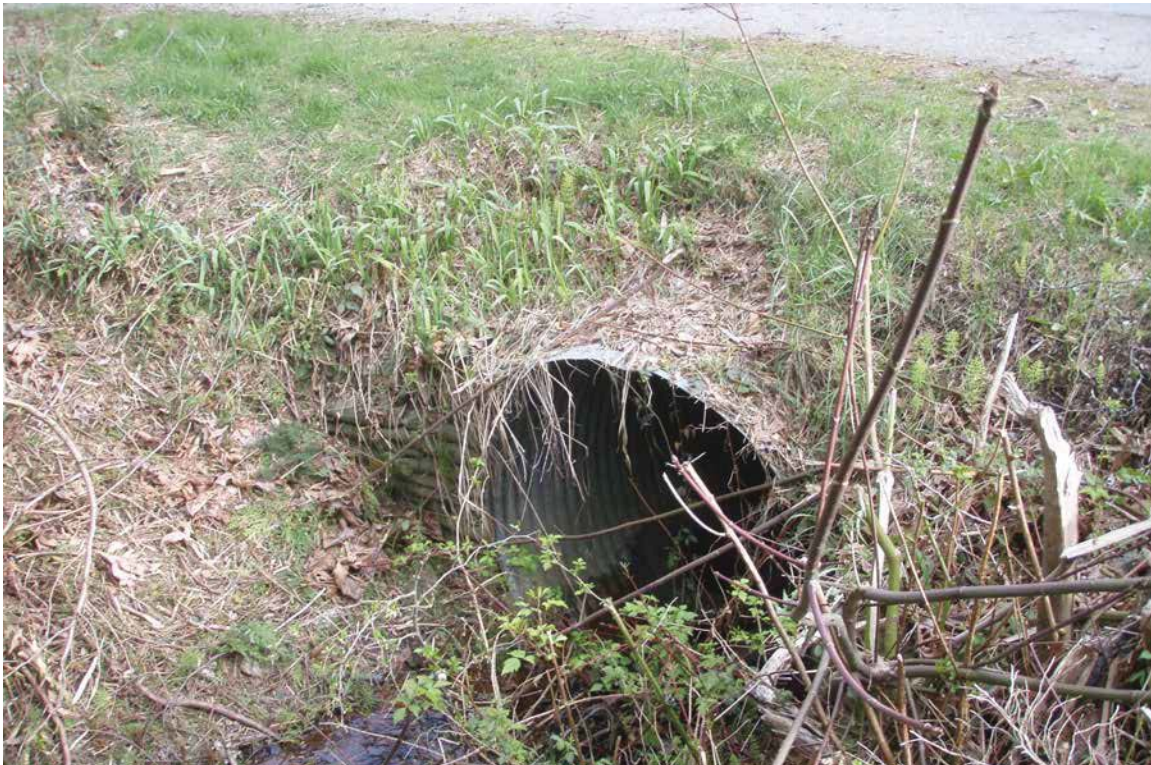
Photo 11 Typical drainage structure in Highway 101
