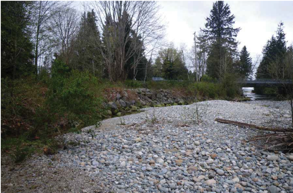
Photo 9 Looking downstream at Highway 101 bridge and riprap on left bank
