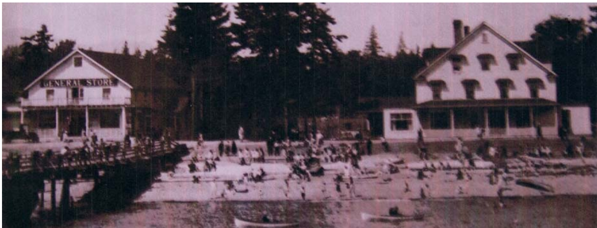
The Sechelt Hotel and General Store are examples of a combination of historic and transferable architectural elements suitable for contemporary building design. Large gable facades have window components arranged in a tiered affect, mirroring the decreasing square footage of upper level stories within the gable. Covered porches, both sloped and as upper level decks, provide protection from the weather and outdoor access to temperate winter climates. Additional gable and shed dormers break up the larger massing of multiple story buildings.
