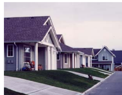
Ensure a variety of building forms, thus reducing uniformity – i.e., not the 'cookie-cutter' approach used in West Sechelt.
