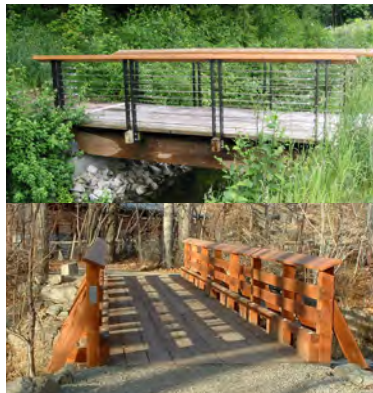
Timber and steel pedestrian bridges
