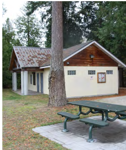
Hackett Park washroom improvements, Sechelt Village
