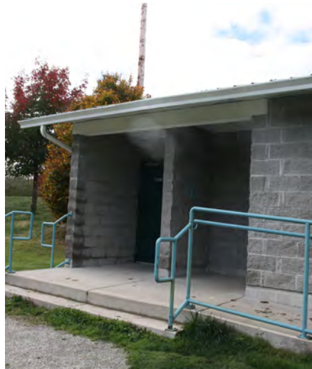
Kinnikinnick Park washroom improvements, West Porpoise Bay
