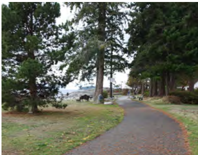
Trail paving upgrades, Snickett Park, Sechelt Village
