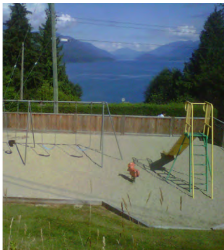
Tot Park is in a central location. The playground will require upgrades in the coming years and there may be opportunities to consider overall park improvements and potential expansion.
