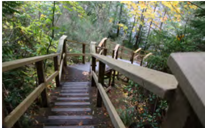
Stair access upgrade, Chapman Creek Trail, Selma Park / Davis Bay / Wilson Creek
