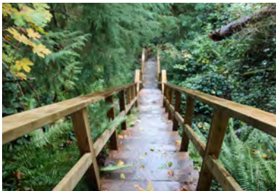
Porpoise Beach Access stair upgrade, Sandy Hook
