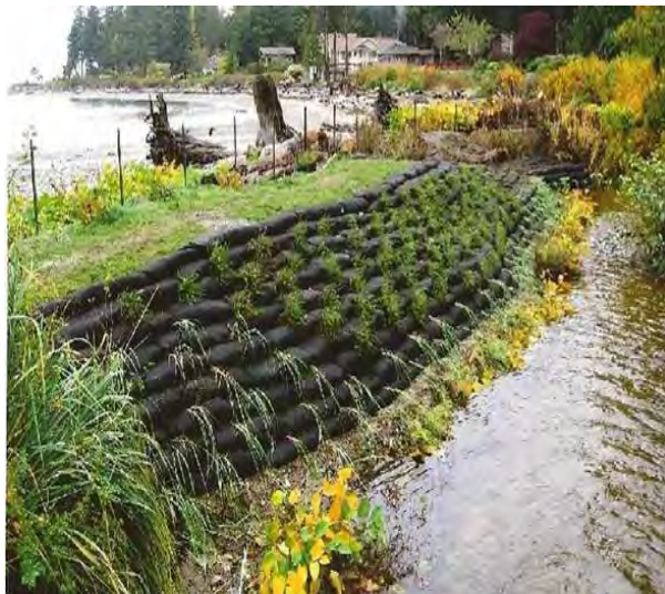
✔ Soft shoreline protection approaches can restore habitat values as well as protect upland property from wave action and erosion (Roberts Creek)
