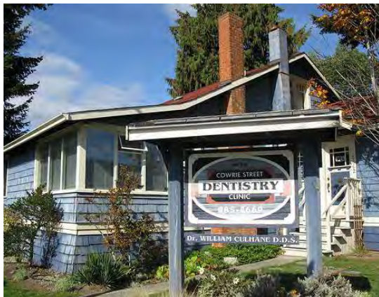
✓ Adaptive reuse of older buildings creates character and a sense of place in the Downtown.
