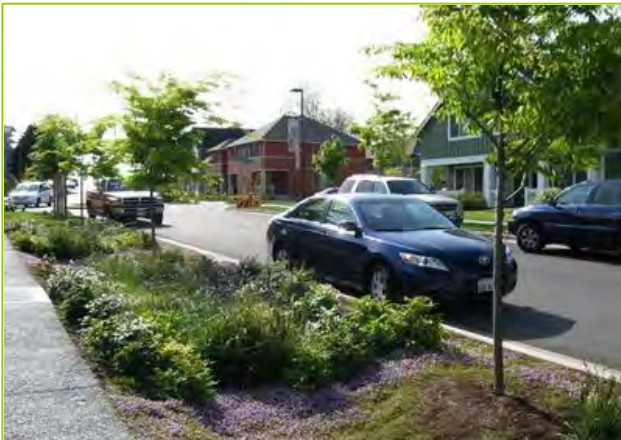
Planted swales provide a landscaped alternative to storm sewers, capturing non-peak rainwater flows. Separated sidewalks encourage pedestrian use
