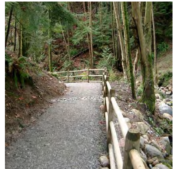
✔ Trails moved back from the stream edge creates safer trails and allows restoration of streamside habitat.
